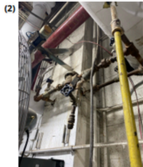
Tag 82 Created: Tue, 4/30/2024 Steam trap on Main Steam line, drip trap, cold.
